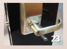
a strong resemblance to Mul-T-Lock high security keys. Along with the keys, you get an interesting key ring magnet that will shortly be demonstrated. The magnet sticks to the figure 8 outline on the front surface of the outside lever handle (photo 23). Presto... and you remove a figure 8 shaped metal plate (photo 24),
