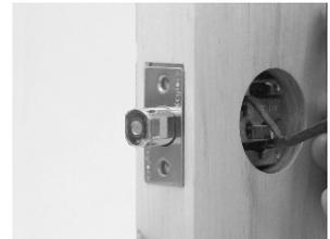
**NOTE:** If the screws are tightened down too much it puts pressure on the tail piece and then on the motor, which will cause the bolt to move slowly.
