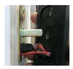
6) Install inside unit onto door, making sure that the spring does not fall out when unit is placed upright and onto the spindle.
