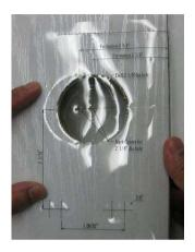
4) Mark the two, 3/8" holes that you cut out of the installation template on the door (with a magic marker).
