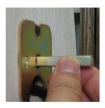
2) Insert spring into inside unit's square hole. VERY IMPORTANT
