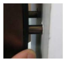
6) Insert outside unit onto the door, making sure that the two middle fixing posts fit into the two holes in the latch and the two bottom fixing posts fit perfectly into the two 3/8" holes.
