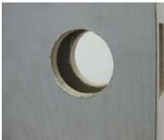
2) Cut out the two, 3/8" holes on the Installation Template that correspond to your existing backset (2 3/8" or 2 3/4").
