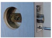
3) Screw the included strike plate into the door jamb.
